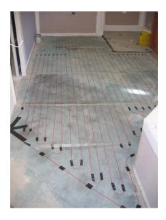
Run the cable around to the opposite side of the heated space, then zig zag the cable back towards the termination point sticking down at the ends only until you are satisfied that reasonably even spacing is achieved. Then apply further strips of tape across the runs at about 400mm spacing. If a floor sensor is used, the sensing tip should be positioned mid way be-
