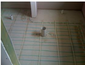
Unroll the cable rather than pulling it sideways in loops, as this will form twists. Take care not to apply unnecessary tension at any time, especially at the end joins. When nearing the end, you may find it necessary to make minor adjustment to spacings in order to finish up where you intended.
